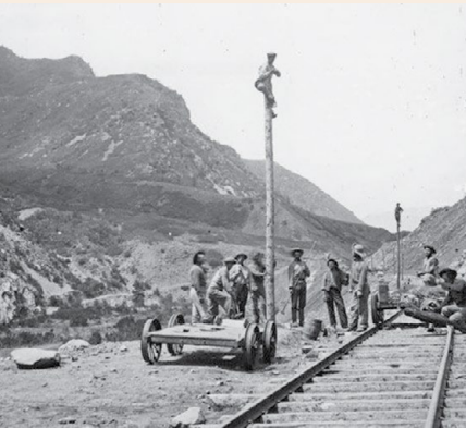
The first pole of the transcontinental telegraph was placed in July of 1861, and, miraculously, it was completed just a few months later with two thousand miles of single-strand wire and more than twenty-seven thousand poles.
