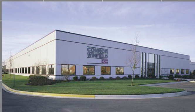
Manufacturing Facility, 2359 Diehl Rd, Aurora, IL
